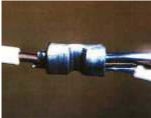
**AMP TYCO COPALUM Copper-to-Aluminum Pigtailing** Use the special AMP (now TYCO) COPALUM high pressure crimp connector and special tool to connect short copper wires to *every aluminum wire end* in the building, reconnecting the copper to the various devices (outlets, switches, lights) and splices.
