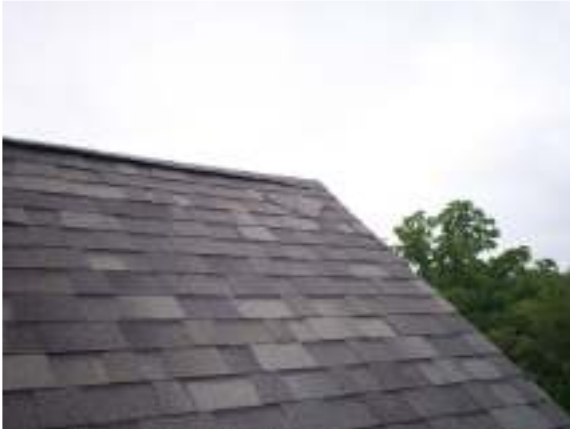
Loose shingle tab noted over the master bedroom area, recommend this tab be re-secured. The flashing over the front porch should be re-secured.
