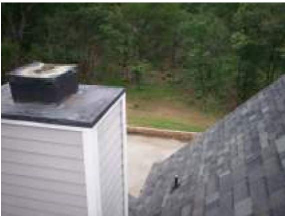
Chimney height does not appear adequate per current industry standards (Code) to ensure proper draft of fireplace. The chimney should extend at least three (3) feet above the point passing
