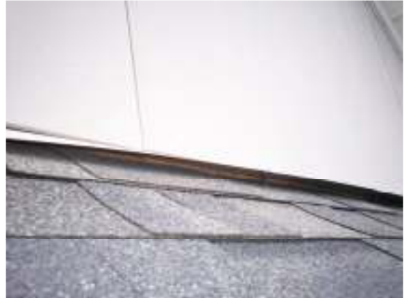
Loose shingle tab noted over the master bedroom area, recommend this tab be re-secured. The flashing over the front porch should be re-secured.
