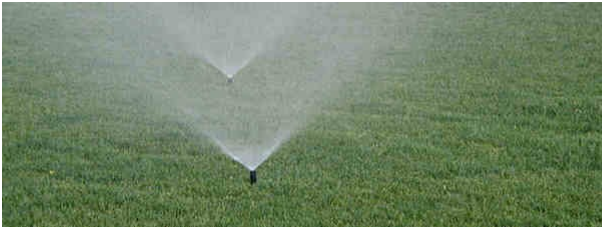
Spray-Type Sprinkler Heads
